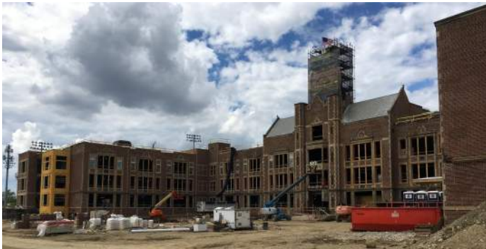
Courtyard Wood Window Replacement
