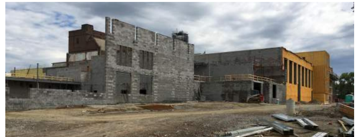
Area B Spray Foam & Area C Masonry
